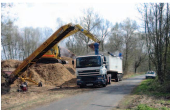
Large amounts of woodchip like this can be used for energy generation; smaller amounts can sometimes be used for path surfacing or mulch
